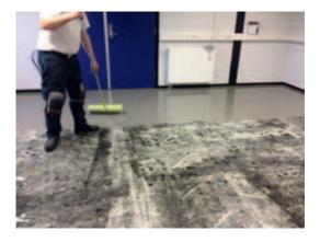
UZIN NC 163 has been developed specifically for the renovation sector and can also be applied directly and effortlessly onto sound, well bonded and waterproof adhesive residues. It is easy to install using a smoothing trowel or using the raking method. The powder disintegrates quickly and without lumps and the excellent flow properties always represent a great basis for any subsequent work. This applies both to new construction or old substrates in renovation work.
